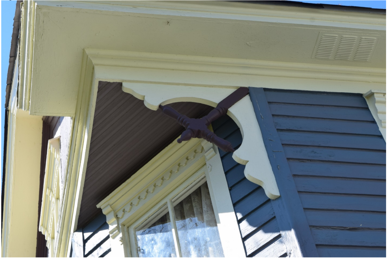
Fig. 4: Bracket under Front Gable
