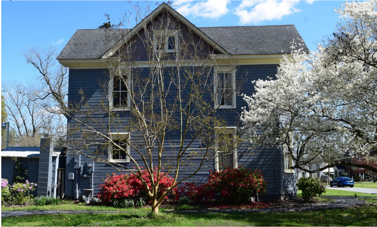
Fig. 10: Molded drip edge, sawtooth ornament and scrolled, console like brackets
