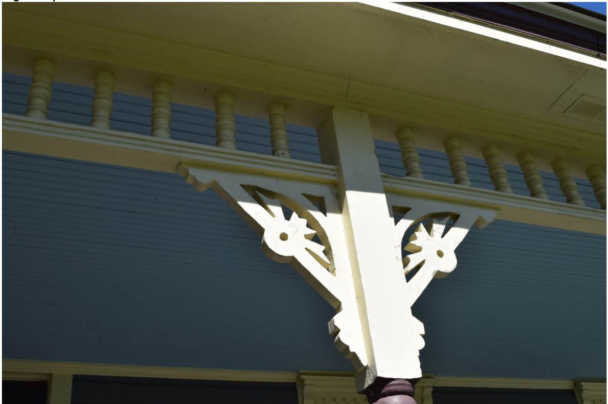
Fig. 7: Spindle Frieze and Brackets
