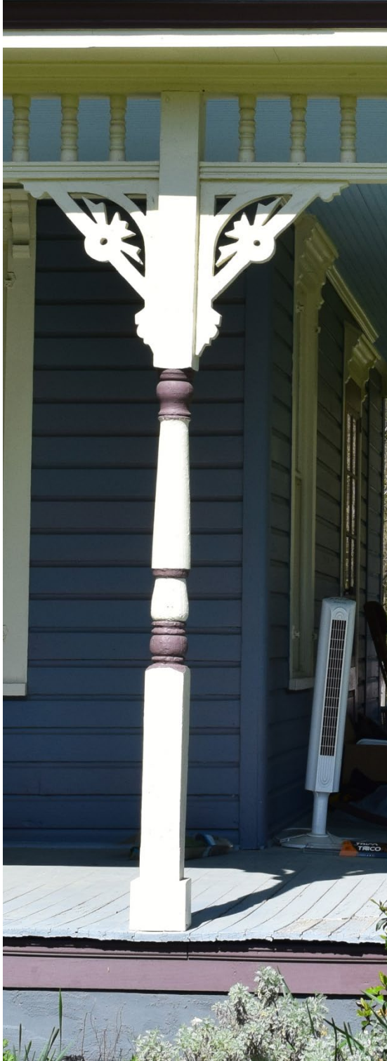
Fig. 8: Turned Porch Spindles, Porch Floor and Trim
